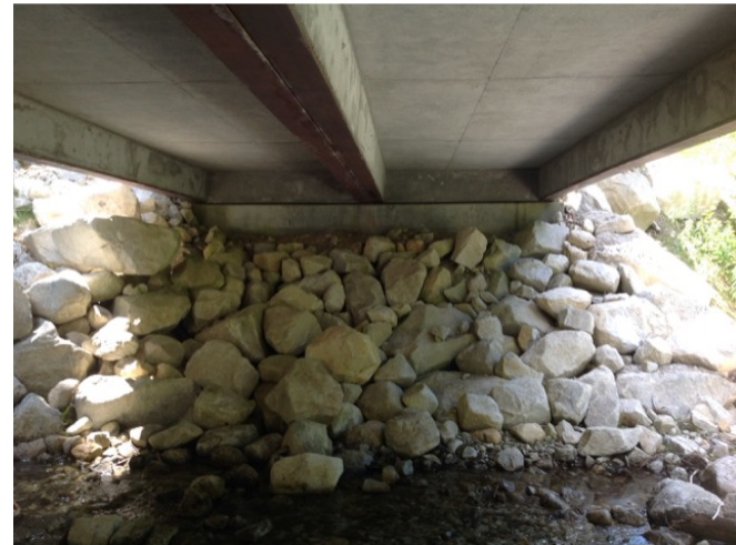
Left Bank Abutment when facing downstream
