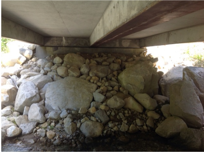
Right Bank Abutment when facing downstream
